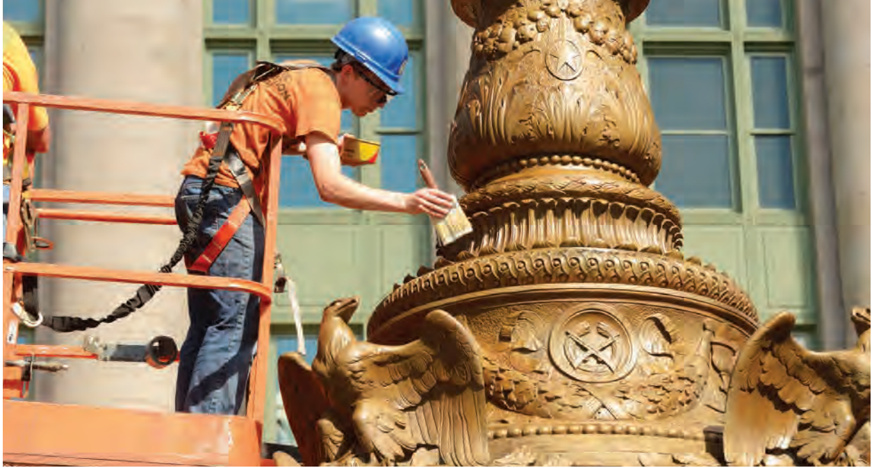
Preservation student Edward Harthorn of St. Paul applies a final coat of paste wax over the newly refinished Soldiers and Sailors Monument in Duluth.
